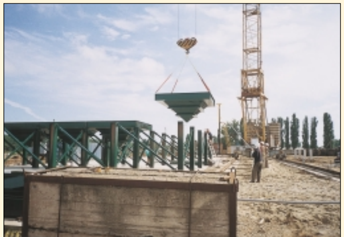
Erection of silo for seed corn
