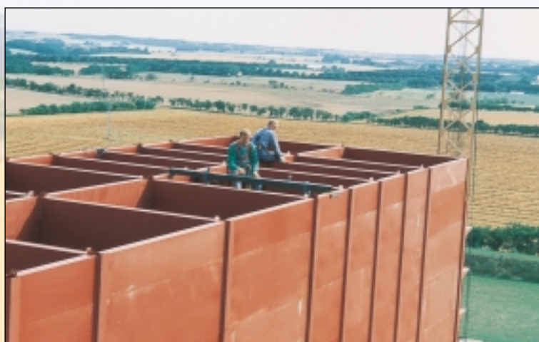
Face plate silo for feedstuff
