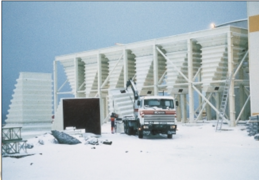
Substructure and silo discharge hoppers for storage of raw material for fish feed, 500 km north of the polar circle
