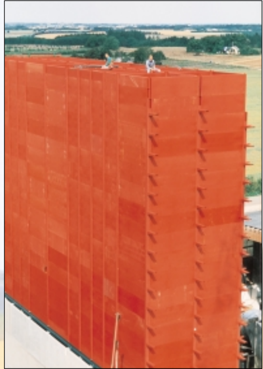
Face plate silo for feedstuff
