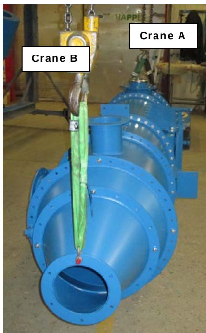
Fig. 3: Filter erection – continued as vertical lift. Crane A: 2 straps attached as shown in fig. 1. Crane B: Slowly raise filter to vertical.
